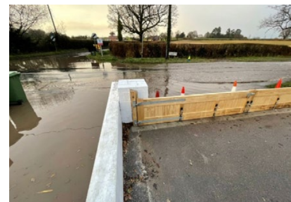
The picture shows the flood barrier in action, successfully resisting a recent flood event.
